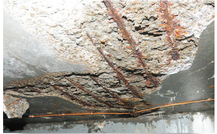
Fig. 4: Corrosion damage at floor slab
