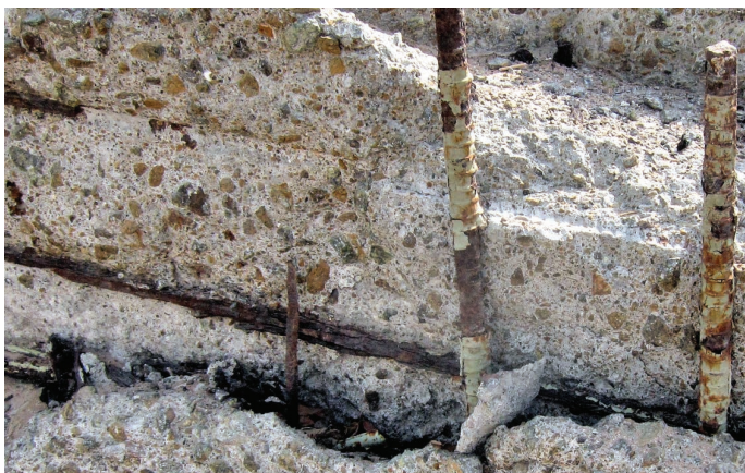
Fig. 5: Corrosion on coated reinforcing steel at a quay wall
