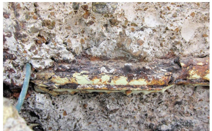
Fig. 6: Corrosion on coated reinforcing steel
